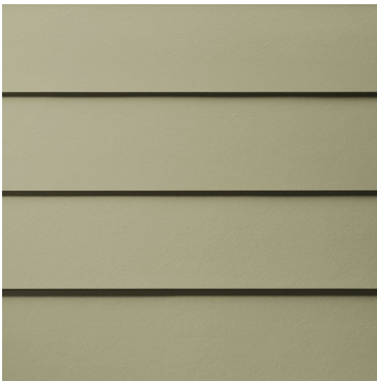
YES. Cementitious siding for should resemble historic wood siding as closely as possible in width and reveal.
