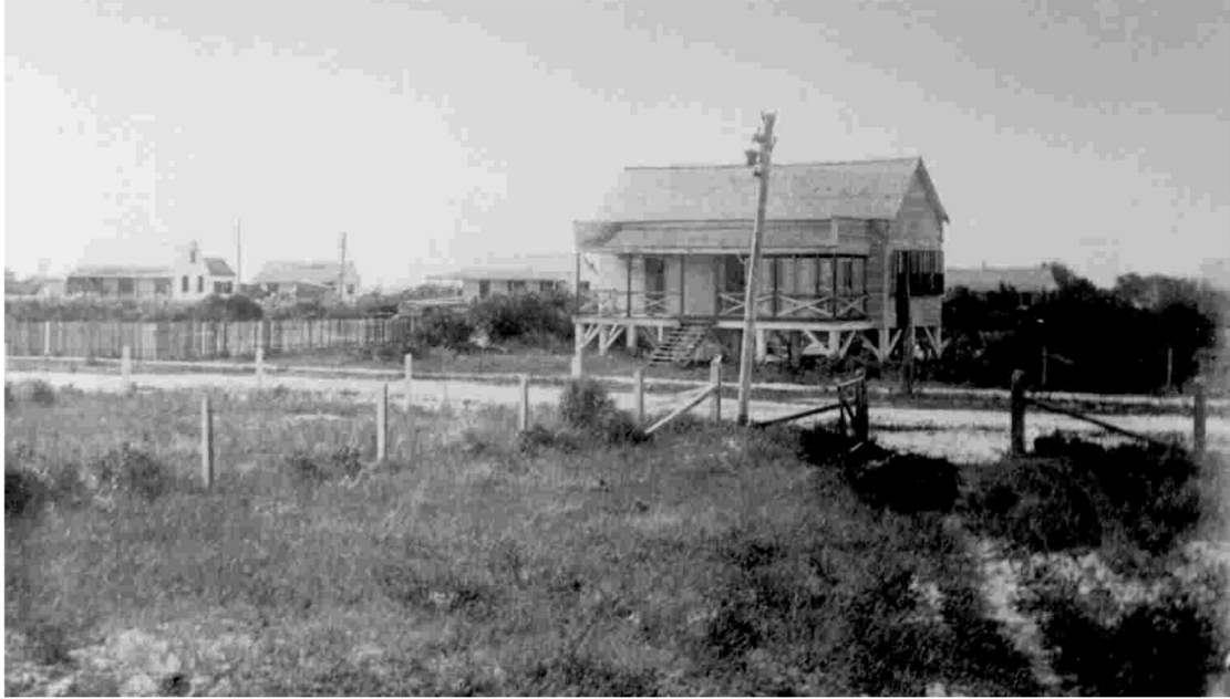
This photograph shows a one-story vernacular dwelling ca. 1900 described as the “Gibbes” House on Sullivan’s Island. It is representative of the typical one-story houses with front porches. (Courtesy of the Historic Charleston Foundation Archives).
