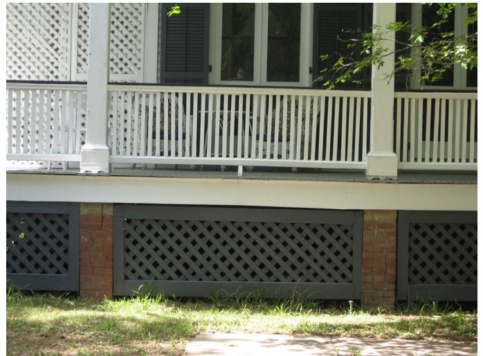
These traditional diagonal lattice panels are appropriately placed between the porch foundation piers at 1744 Iron Avenue.
