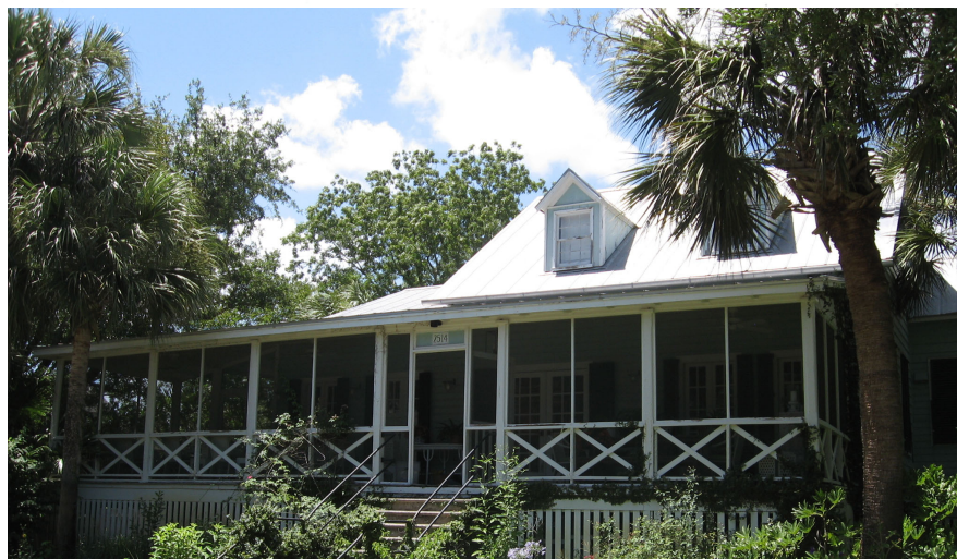
Another common typology is a one and one-half story cottage with an "L" shaped porch, (2504 G'on Avenue).
