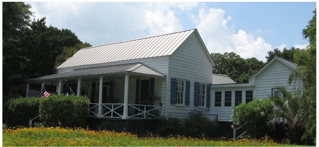
Many of the historic homes were enlarged over time with lateral or rear wings as at 1808 I'on Avenue.
