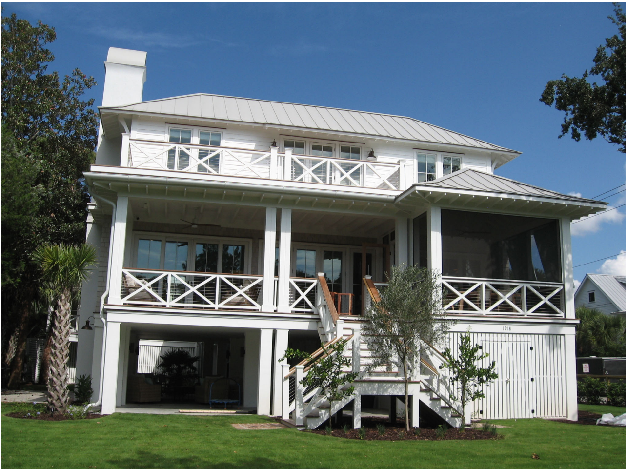
The dwelling at 1918 I'on Avenue was built in 2023 and designed to meet the Town's Design Flood Elevation (DFE). It reflects the historic vernacular forms of the island with its hipped roof, siding materials, and railing design.
