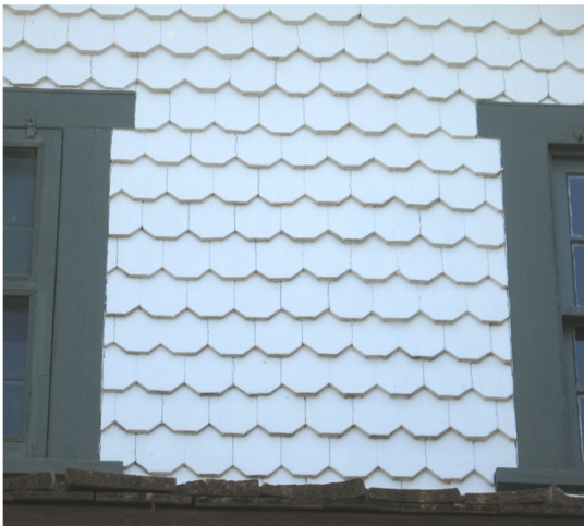
Decorative materials such as wood shingles should be preserved and maintained (1815 I'on Avenue).
