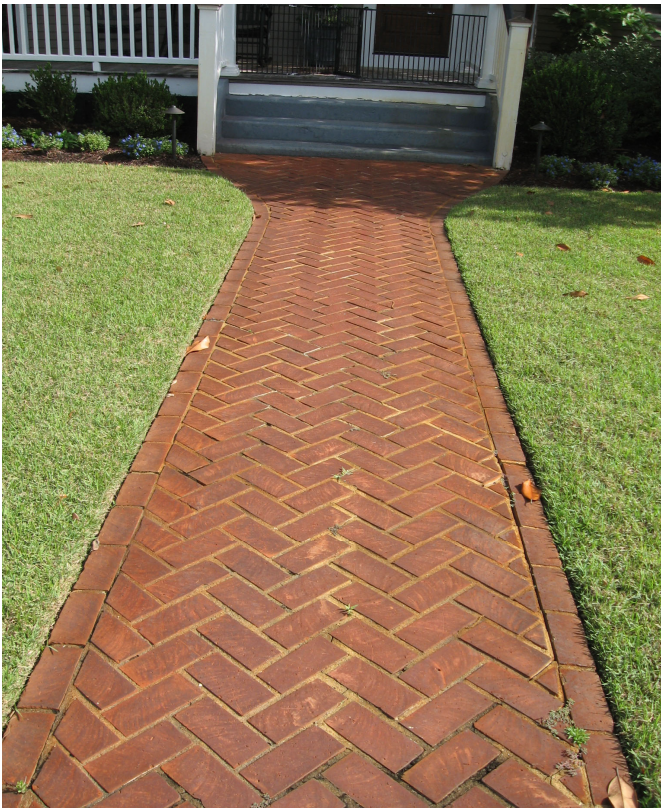
Brick walkways from the early- to -mid-20th century should be preserved and maintained as at 1722 Middle Street.
