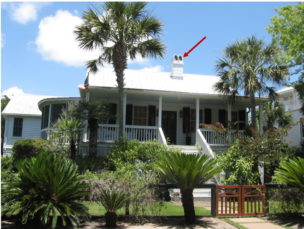
Elevation projects should have the chimneys preserved and elevated with the dwelling as at 950 Middle Street.
