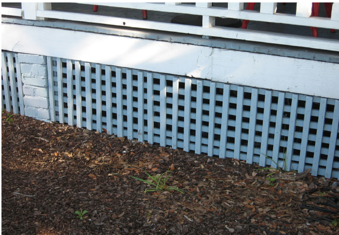
Lattice panels are appropriate treatments for screening between brick piers (2120 Middle Street).
