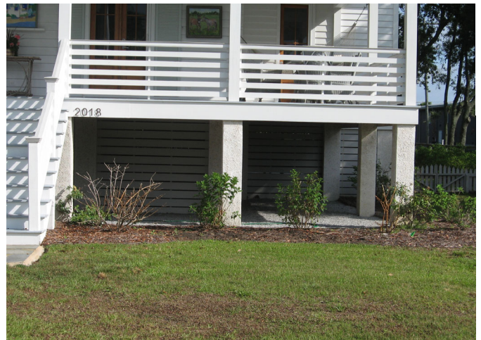
These stuccoed concrete piers are appropriate for the dwelling and are aligned with the porch columns above (2018 Middle Street).
