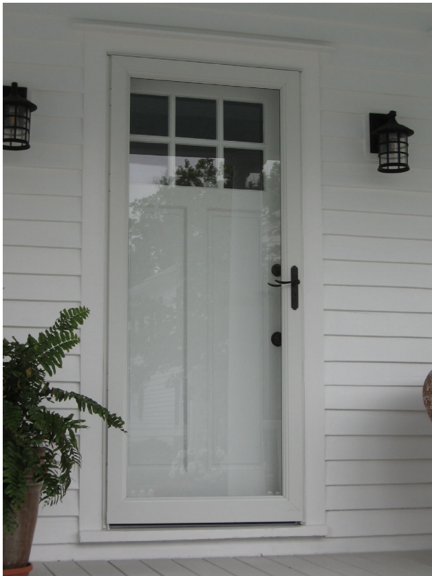
YES- Storm doors should be unobtrusive and blend with the historic door as in this example.
