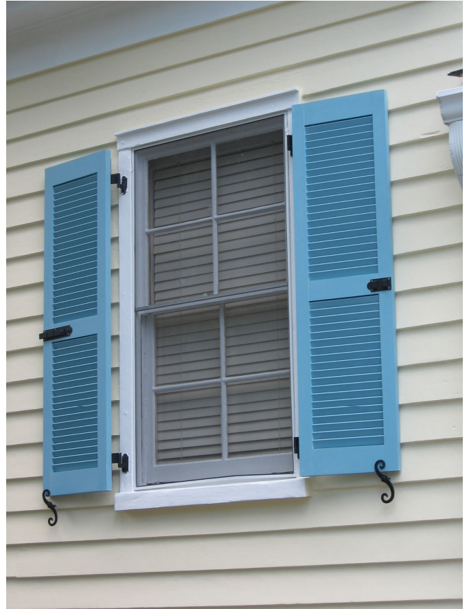
The most common types of shutters in the historic districts are raised panel designs (1726 Middle Street, left) and louvered designs (2424 Middle Street, right).
