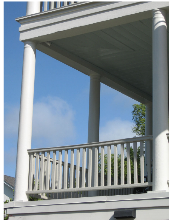
By the early twentieth century, porch columns were often designed in classical styles including Tuscan, as at 1808 Middle Street.
