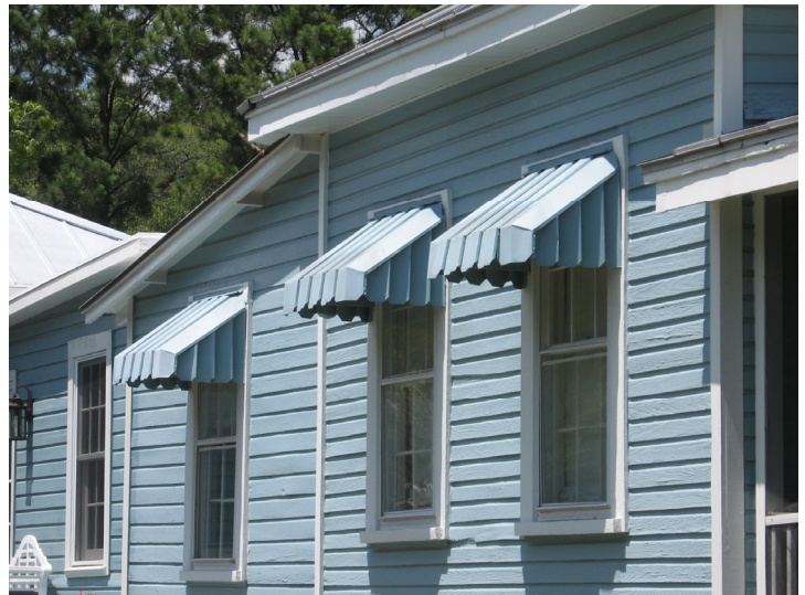
Appropriate metal awnings at 2614 Myrtle Street.
