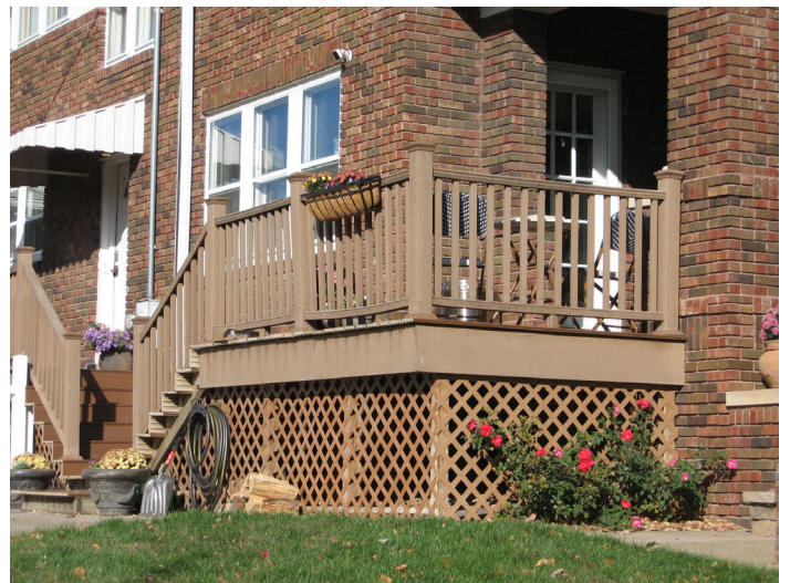
YES: This deck is appropriately sited at the rear entrance, has square balusters and lattice panels to enclose the foundation.
