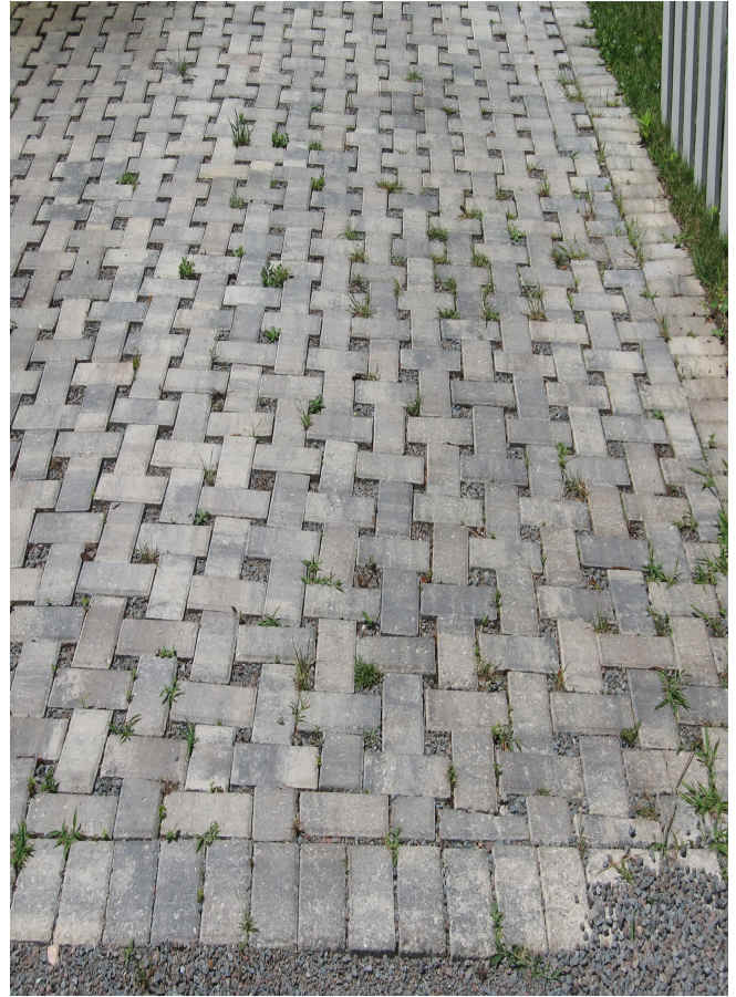
Driveways should be of permeable paving materials to allow for water absorption. At left is a driveway composed largely of gravel at 2061 Pettigrew Street. At right is a driveway at 2614 Myrtle Street of interlocking concrete pavers which helps to decrease water runoff.
