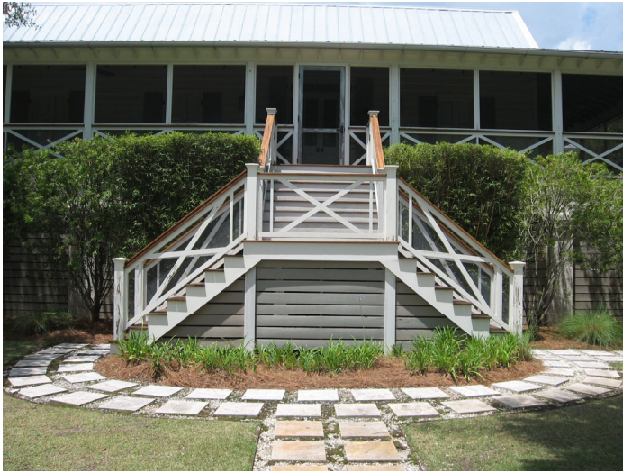
Example of a center/linear split staircase for a high increase building elevation project (2408 I'on Avenue).
