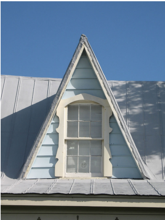
The dwelling at 2002 Middle Street features a gable dormer and decorative window surround at the roofline.
