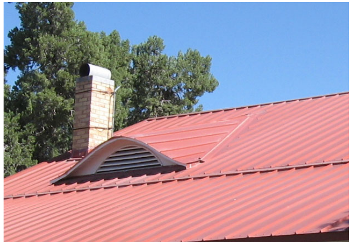
NO - Metal roofs which do not have traditional standing seam profiles and spacing are not appropriate.
