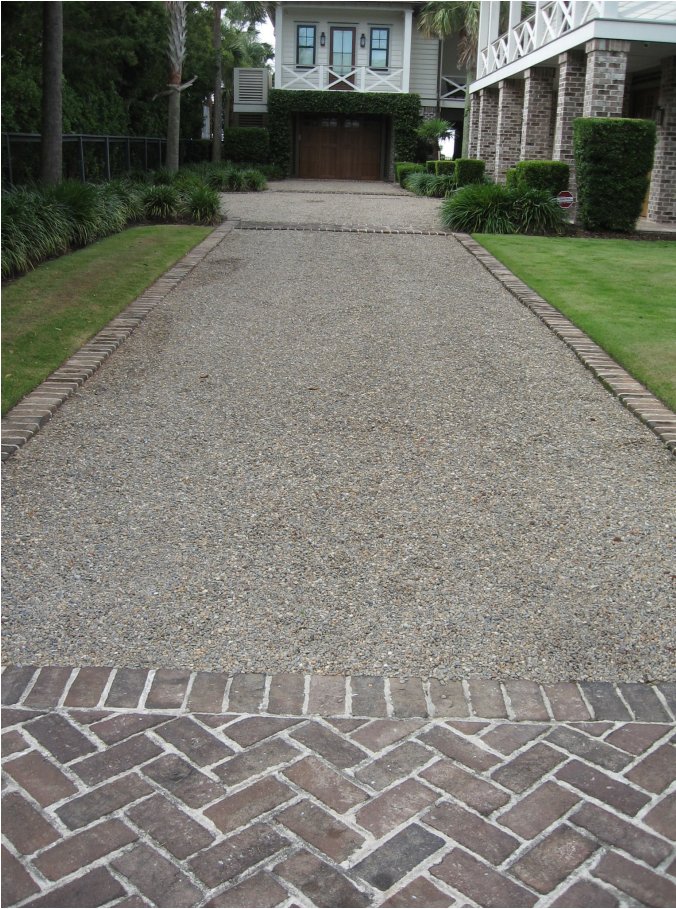
Driveways should be of permeable paving materials to allow for water absorption. At left is a driveway composed largely of gravel at 2061 Pettigrew Street. At right is a driveway at 2614 Myrtle Street of interlocking concrete pavers which helps to decrease water runoff.
