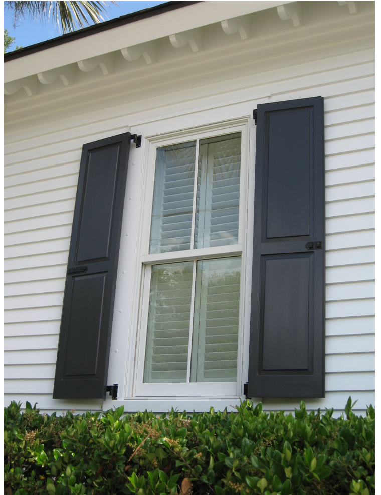
The two-over-two sash window at 1514 Middle Street is an example of an appropriate aluminum clad wood sash window.
