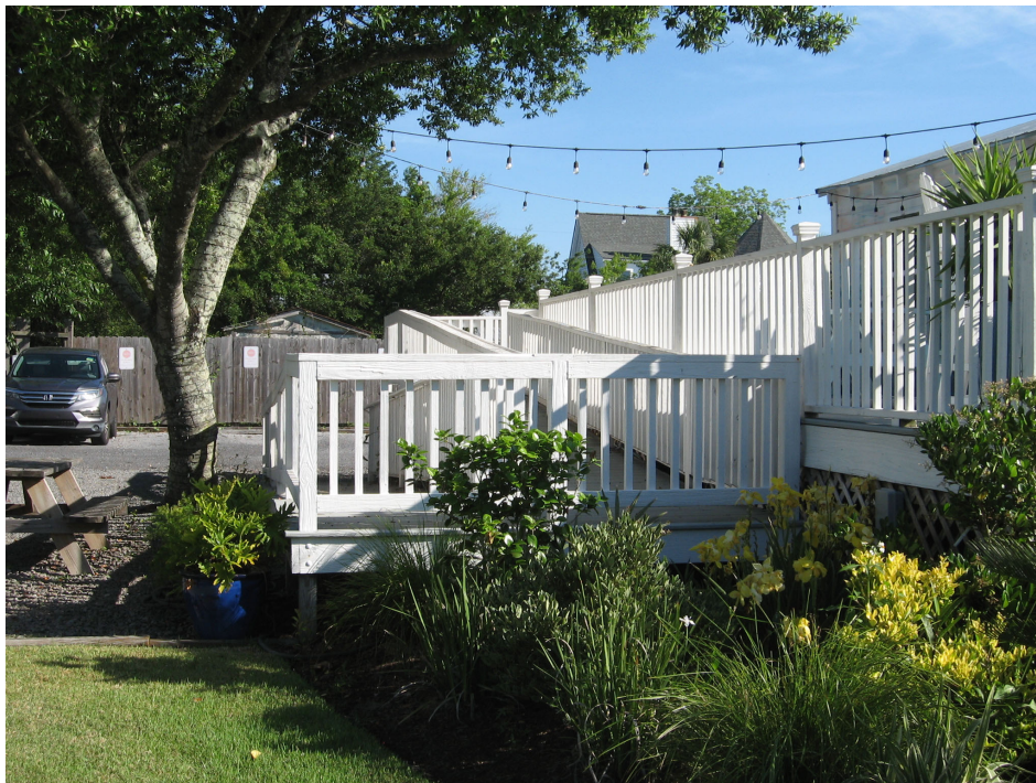
This former dwelling at 2216 Middle Street was converted into commercial use which required an ADA ramp (above). The ramp was sited on a side elevation and its design is in keeping with the porch railing. The ramp is appropriately screened through landscaping (below).
