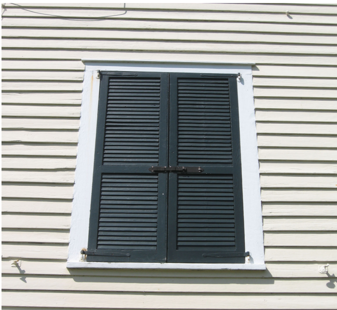
When closed, shutters should cover the window opening to which they are attached (1820 Central Street).
