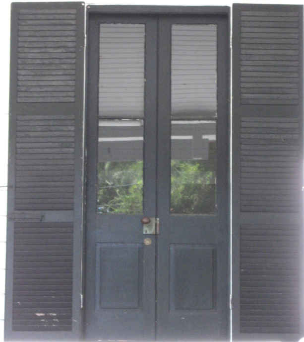
Shutters original or appropriate for an entrance should be preserved and maintained (2662 Jasper Street).
