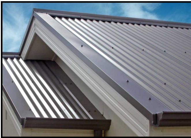
NO - Metal roofs which do not have traditional standing seam profiles and spacing are not appropriate.
