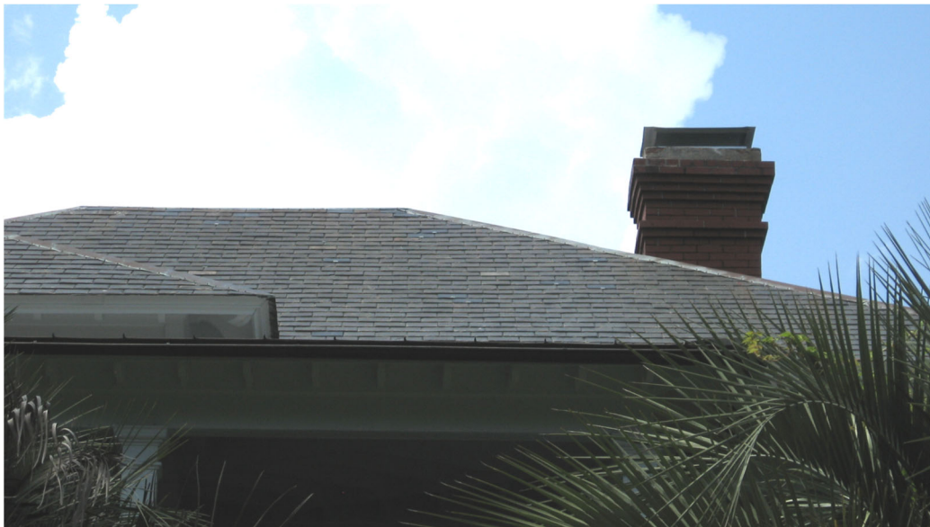
Only a few original slate roofs exist in the historic districts. These can last indefinitely and are important defining features of a property (1760 I'on Avenue).
