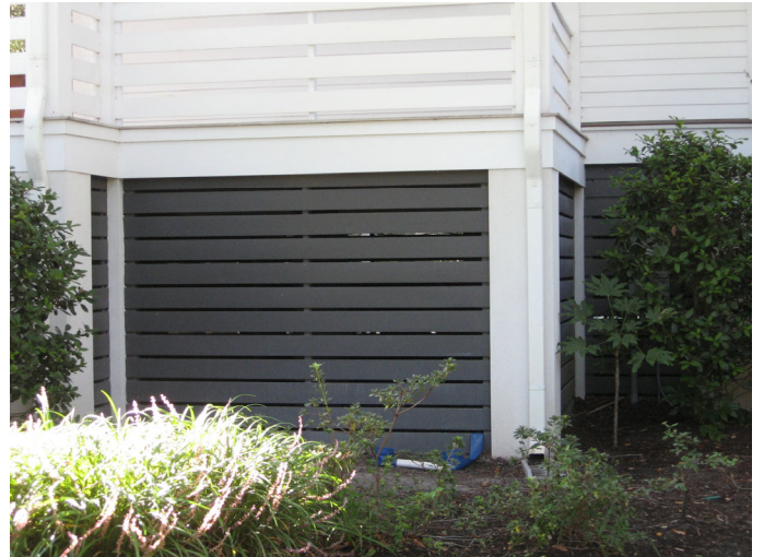
Horizontal slats between foundation piers is also a common design element for elevated houses in the historic districts (2430 Ion Street, top, 2502 Myrtle Avenue, center, and 1607 Middle Street, bottom).
