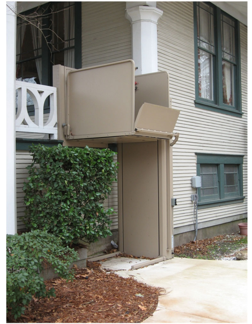
ADA compliance can be achieved for low elevation buildings through adding chair lifts. This example shows an ADA-compliant parking space and a lift screened with landscaping. Only a small section of this porch railing was removed and can be reinstalled when the lift is no longer in use.
