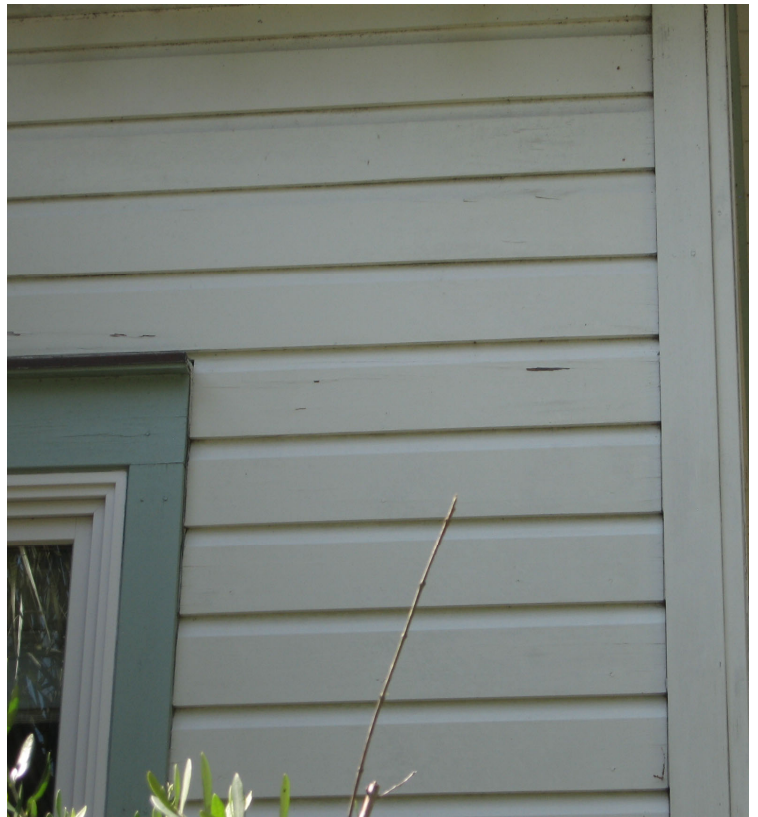
At left is the weatherboard siding at 1754 Central Street which contrasts with the novelty (or drop) siding which has tongue-in-groove boards with concave curves as at 1902 I'on Avenue at right.
