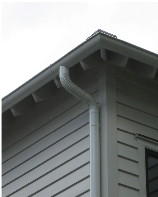
Gutters are recommended to be half-round design with round downspouts, (924 Middle Street, left and 2612 Jasper Street, right).
