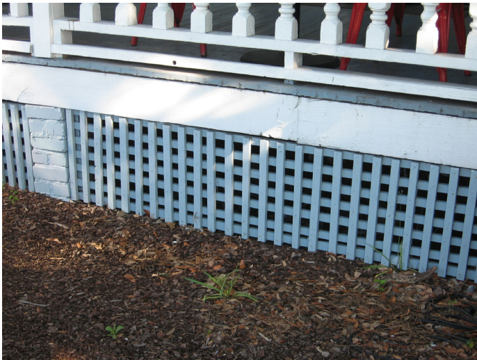
Appropriate vertical and horizontal lattice panels at 2120 Middle Street.
