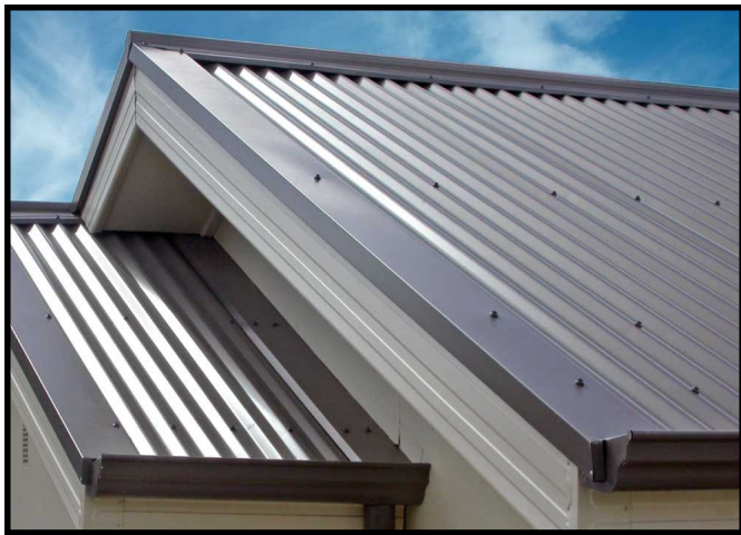
NO - Metal roofs which do not have traditional standing seam profiles and spacing are not appropriate.
