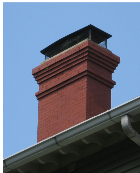
Examples of appropriate chimney caps include the dwelling at 950 Middle Street (left) and the metal chimney cap at 1754 Central Street (right).
