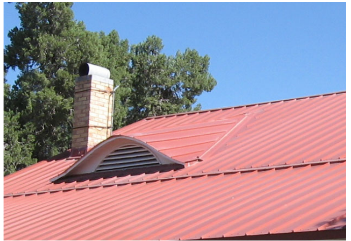
NO - Metal roofs which do not have traditional standing seam profiles and spacing are not appropriate.
