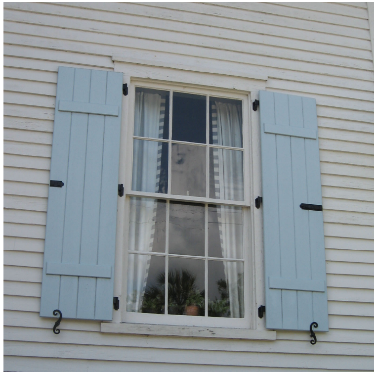
Many appropriate shutter designs are within the historic districts. These vertical board shutters are operable and can be closed to protect the window during storms (312 Station 16 Street).
