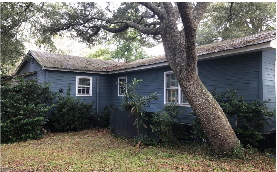
Perspective view of the ell bay, which has vinyl windows and horizontal wood siding.
