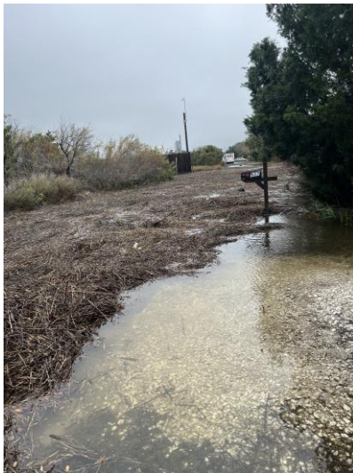
Figure 2 – Flooded Osceola Avenue (near Sta. 9 ½) December 2023
