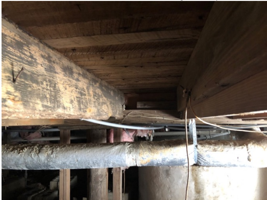
The cistern, foundation, and floor sheathing below bay 3.
