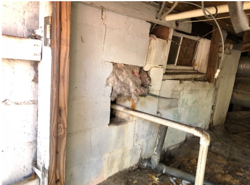
The CMU wall with a basement window is the demarcation between bay 6 and bay 3.
