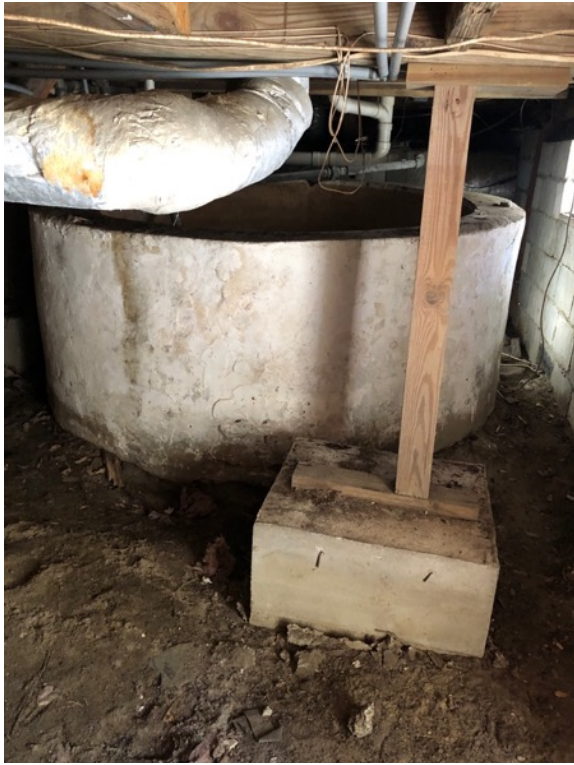
The cistern, foundation, and floor sheathing below bay 3.
