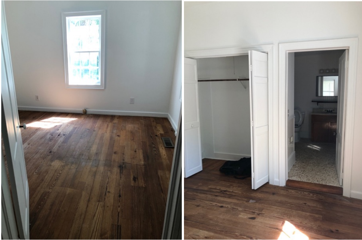
A third bedroom is located off of the living room, to the right. The bedroom is located in bay 1 of the original house. The closet and bathroom are in addition bay 3. Note the historic flooring in the bathroom, and the large threshold to the bathroom where the original back wall of the cottage was located.
