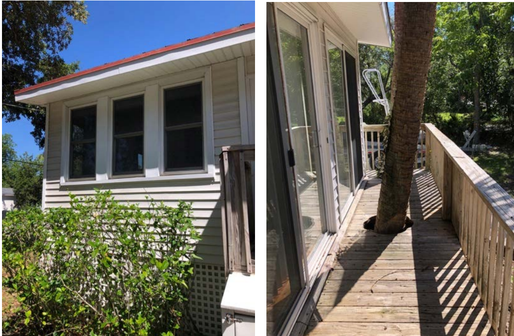
Left: earlier enclosed section of the porch; right: porch enclosure with sliding glass doors.
