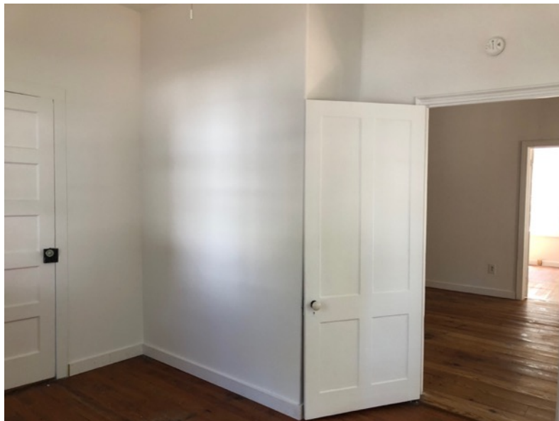
Front bedroom in bay 1, facing the living room. The four panel wood door is historic and retains it ceramic doorknob. The projection pumping into the room is the drywalled chimney box.
