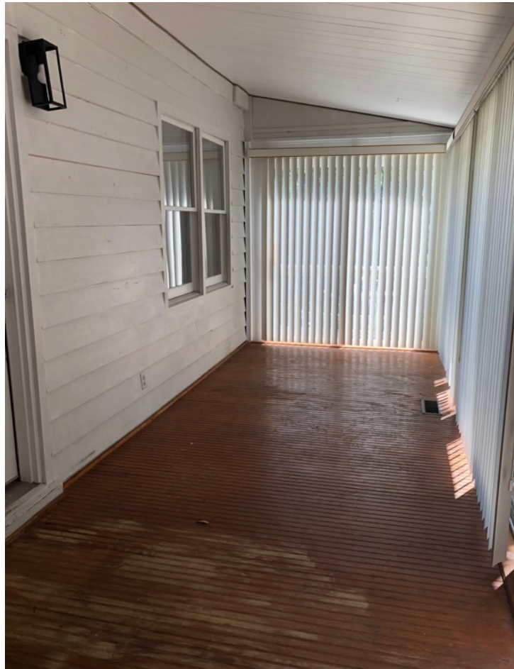
The enclosed front porch, facing west.
