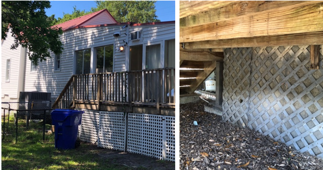
View of the framing below the side deck, showing the solid masonry foundation wall below bay 6.
