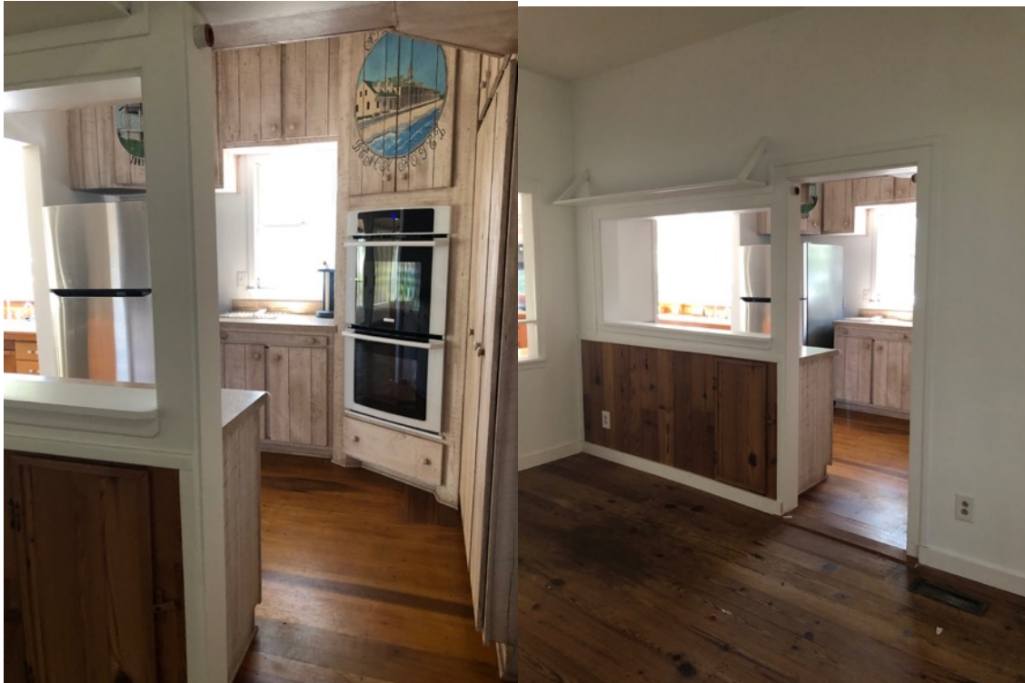
The kitchen (addition bay 3) viewed from the living room. There is no historic material in bay 3, which holds a modern kitchen and bathroom. The former exterior wall was altered with an unglazed opening sometime after the central shed-roofed bay 4 was added.
