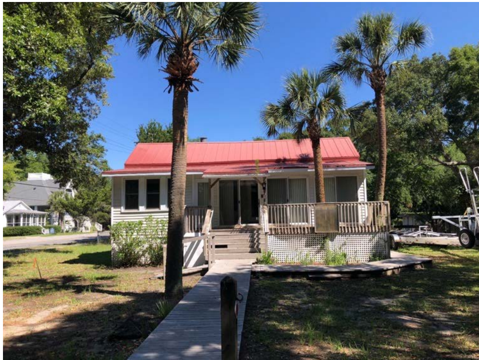
Facade with enclosed porch.
