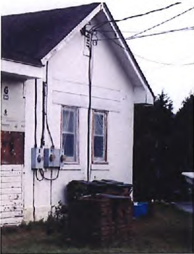
Preparation for vinyl 2002, side view, with further changes to maintain the building with appropriate residential products
