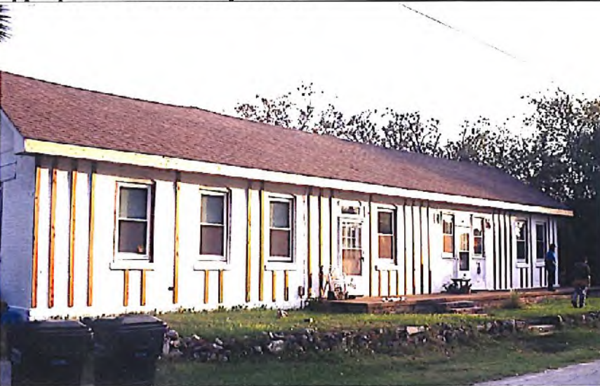
Preparation for vinyl 2002, front view
