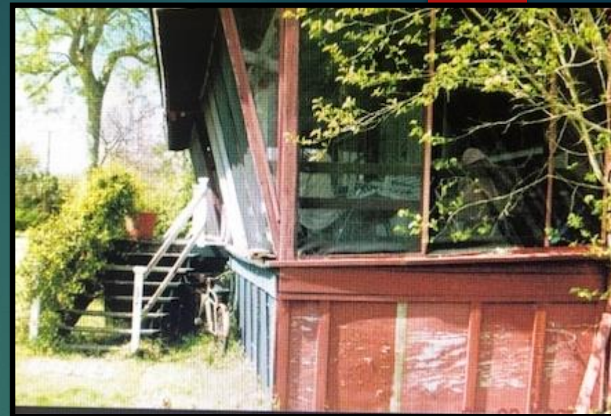
before initial restoration
