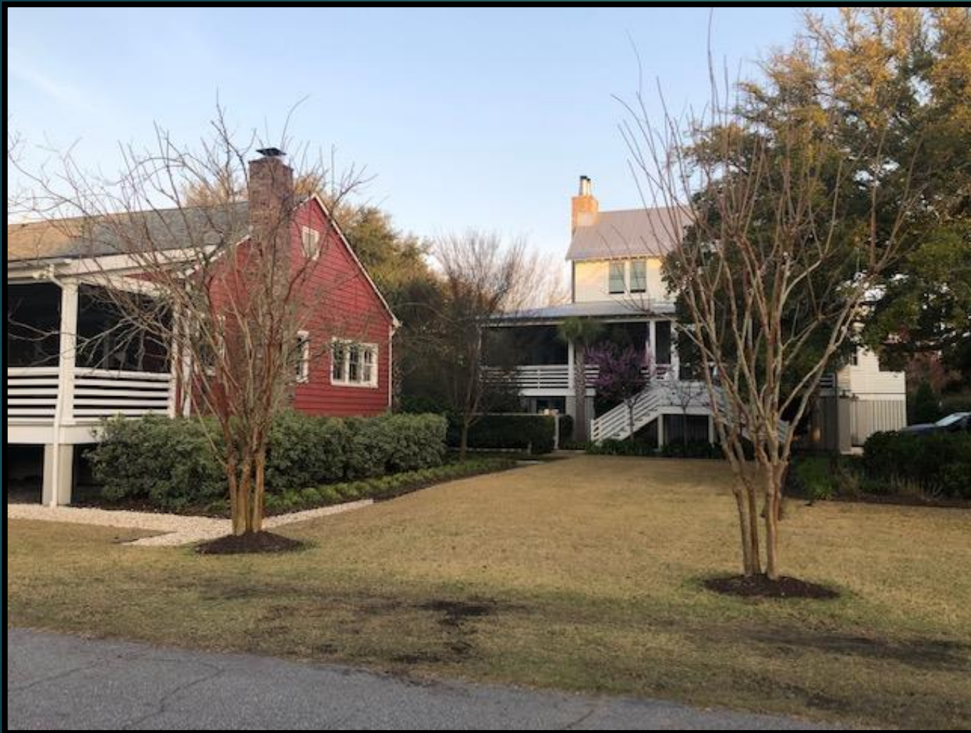
after new construction
